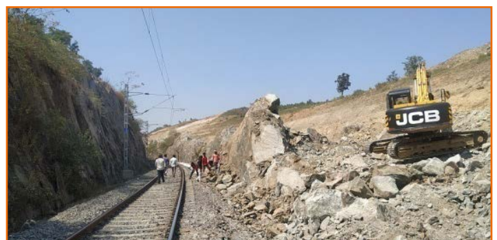
Doubling site of railway line at Karaila-Anpara Section, ECR using controlled blasting
