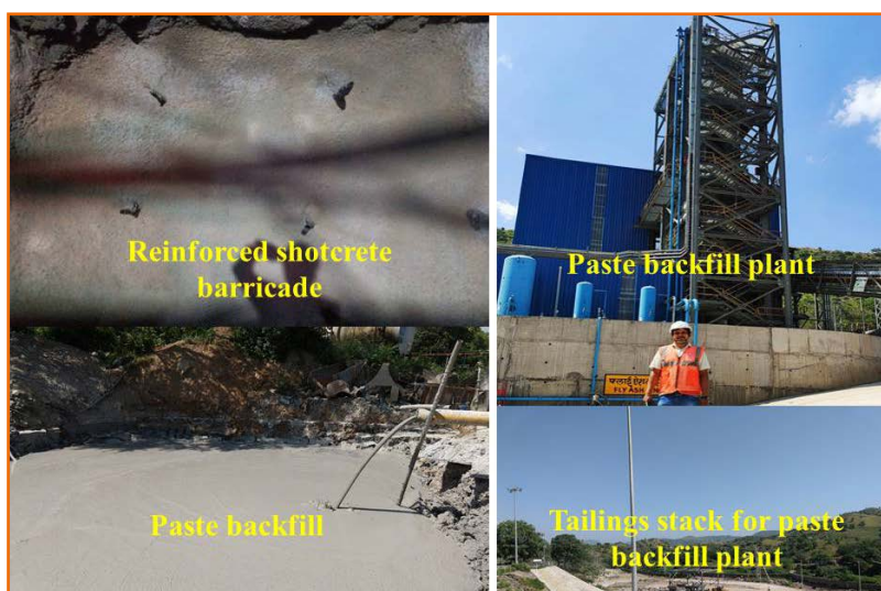
Fig. 5. Paste backfilling in underground metal mines of HZL.
