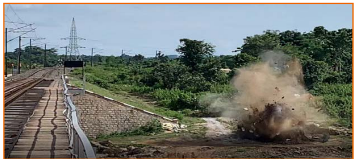
Controlled blast conducted for foundation of 2nd Railway Line bridge pier at Koel river near Bano, Jharkhand, SE Railway
