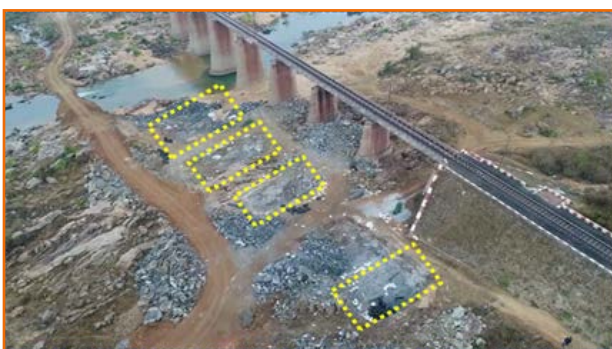
Foundations excavated using controlled blasting for construction of Pier for 2nd Railway Line bridge at Koel river, SE Railway
