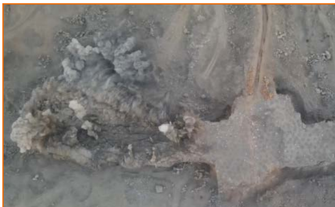
Ulwe Hill for construction of Navi Mumbai International Airport (No. of holes - 620 holes, Rock volume blasted - 1,58,600 m 3 , Explosive used - 78 Tonne)
