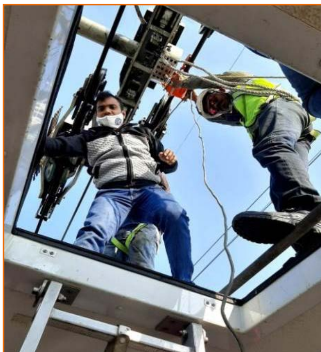
Installed Wire Rope Tester on track ropes of Cable car ropeway at Guwahati, Assam
