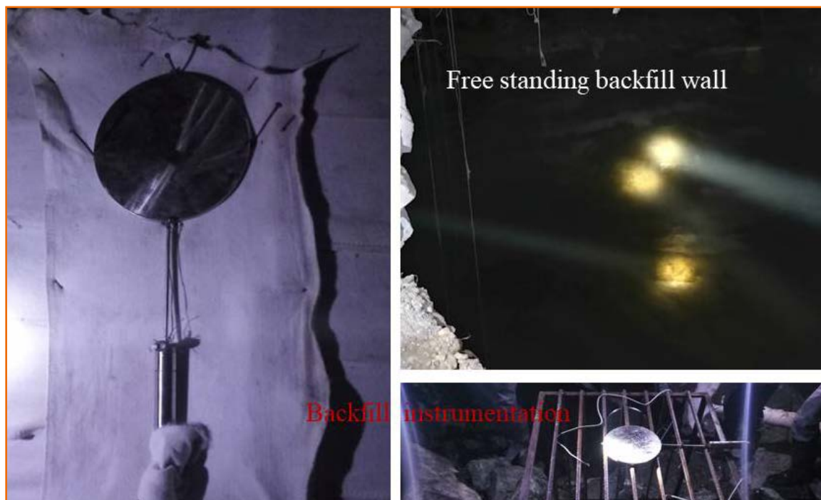
Fig. 4. Backfilling at Mahagiri mines, IMFA with free standing backfill wall and backfill instrumentation.
