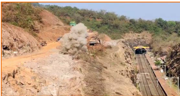
Directional Controlled blasting for flattening of slopes at Ukshi station of Konkan Railway
